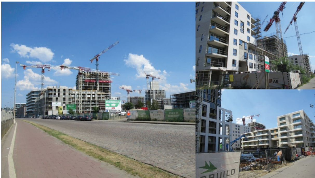
Picture 4 On-going works in Nieuw Zuid Source: UIA Expert
