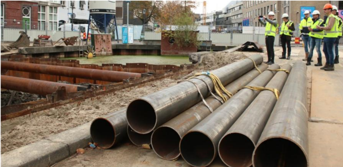
Steel pipes. Image: Birgit Georgi.
