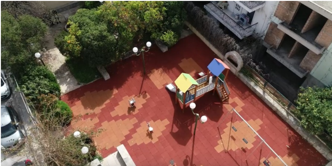
Restoration of Ellis playground in Piraeus.
