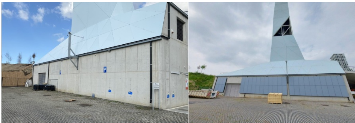
BIPVs on the heatplant, before and after © Ecopower
