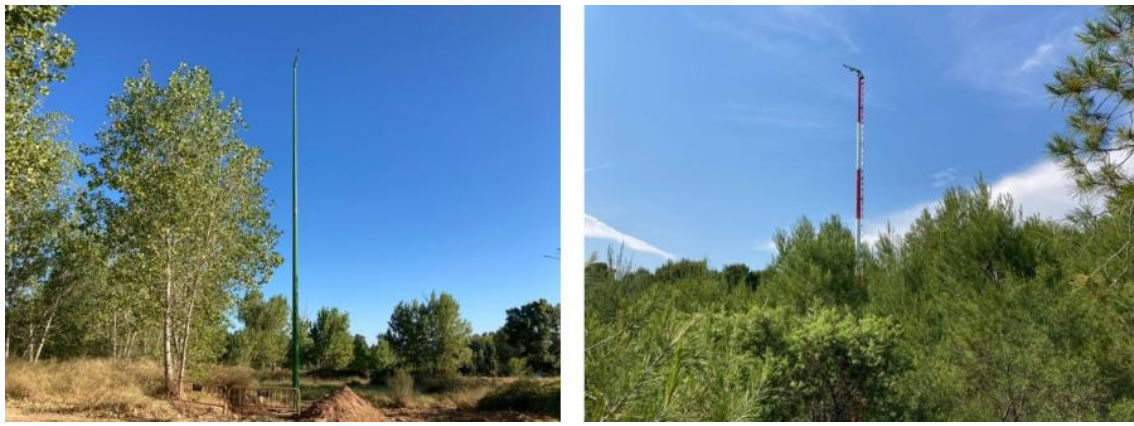
Figure 3. Left: Tower at Masia Traver site, painted in green to achieve landscape integration. Right: Tower at Cañada Sur site, painted in white and red strips in accordance to airport regulations.
