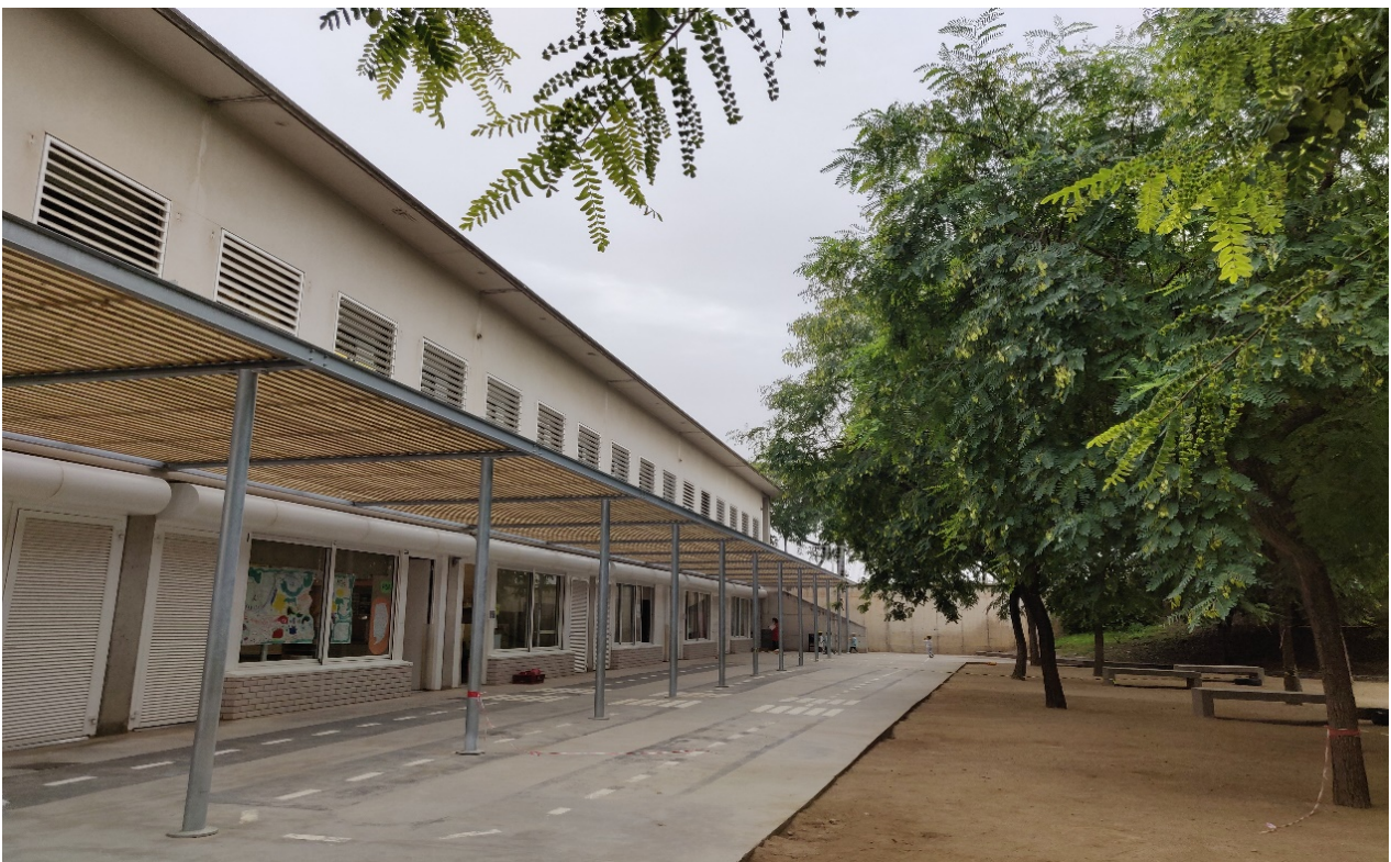
Figure 4. Shading in all classrooms' windows at the Villa Olímpica school has improved indoor temperature conditions and facilitated improved ventilation patterns.
