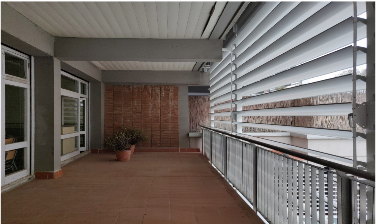
Figure 3. Shading device at the façade of the Poblenou school, also leading to a new working space for the school.
