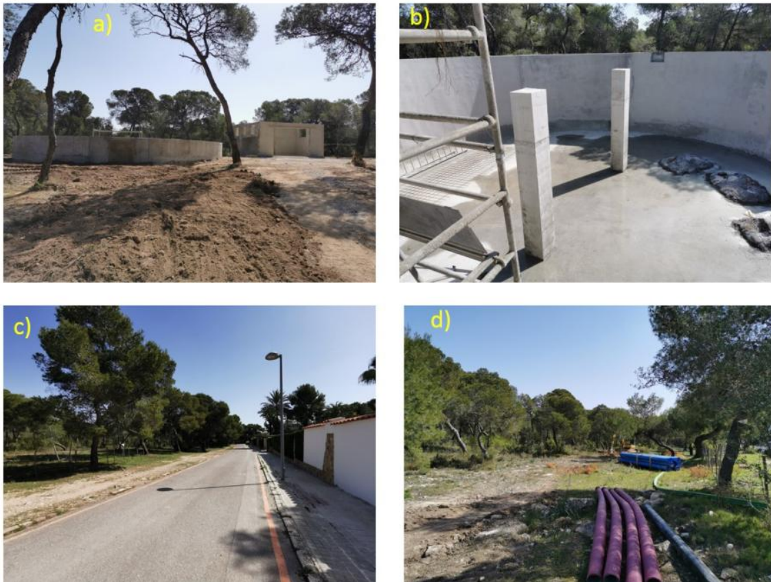
Figure 5. Building works at the Bravo water tank: a) external view; b) internal view of the tank; c) WUI perimeter at “Cañada Norte” settlement in which green fire breaks are being constructed; d) Pipelines ready to be buried to convey water to 6 cannons which will work at a flow rate up to 800 L/min.
