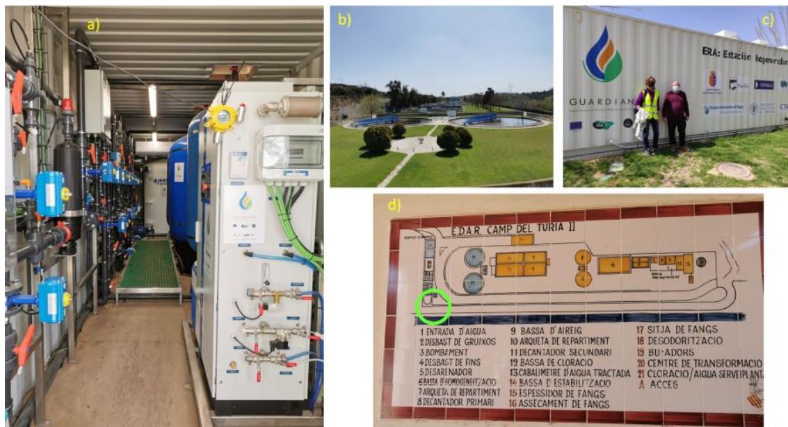
Figure 1. a) The WRP equipment. Look how many compounds integrating a high-tech water treatment process can be put into such small container; b) The WWTP “Camp the Túria II”: waste water engineering environment can be even beautiful! c) the High Cube Container (with prof. F. Hernández (Universitat de València) and myself); d) WWTP sketch in tiles (the green circle is where the WRP is located), difficult to updated it, though!
