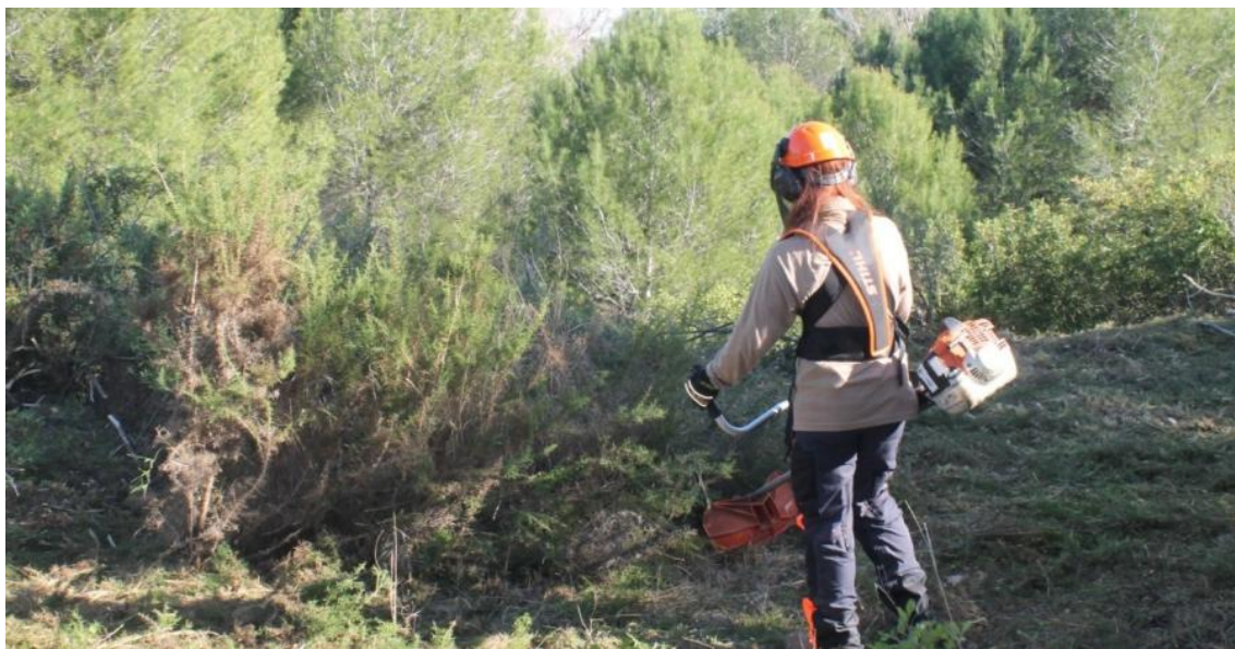
Figure 8. Clearing job performed at La Vallesa forest by MEDI XXI technician. The company has temporarily increased its staff by 10 new members specialized in forest management works.
