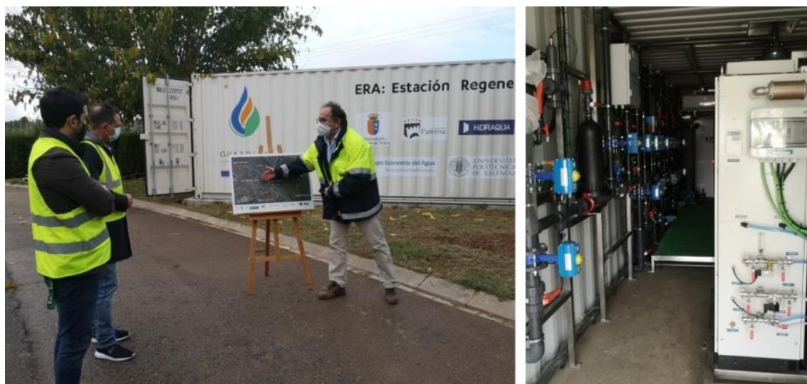
Figure 1. Left: HIDRAQUA engineer briefing end-users on the GUARDIAN water cycle just in front of the just-installed WRP. Right: Water treatment equipment and pipelines constituting the WRP located inside the High Cube container.
