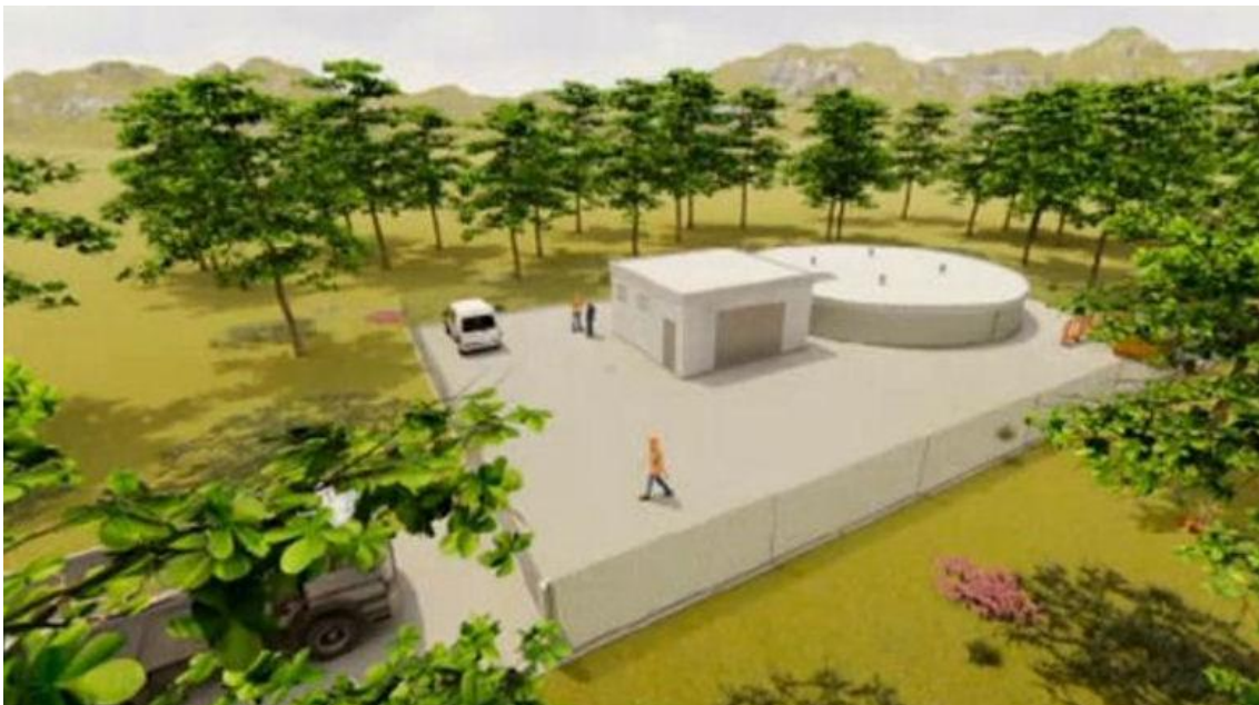
Figure 5. 3D recreation of one of the GUARDIAN water storage tanks. The tank is half-buried (with 1.8 m height above ground). The adjacent control house contains pumping instrumentation and a generator for auxiliary energy supply in case of wildfire.
