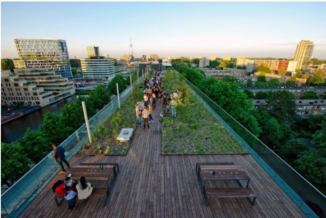
Another view of the De Boel Blue-Green Roof (photo credits: Vesteda)
